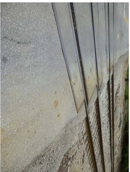
Gaps between the roadway and rail can pose a danger to people walking, biking, or using mobility devices.
