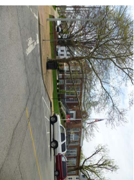
This bumpout in front of the Kirkwood Library helps to narrow the roadway and calm traffic.
