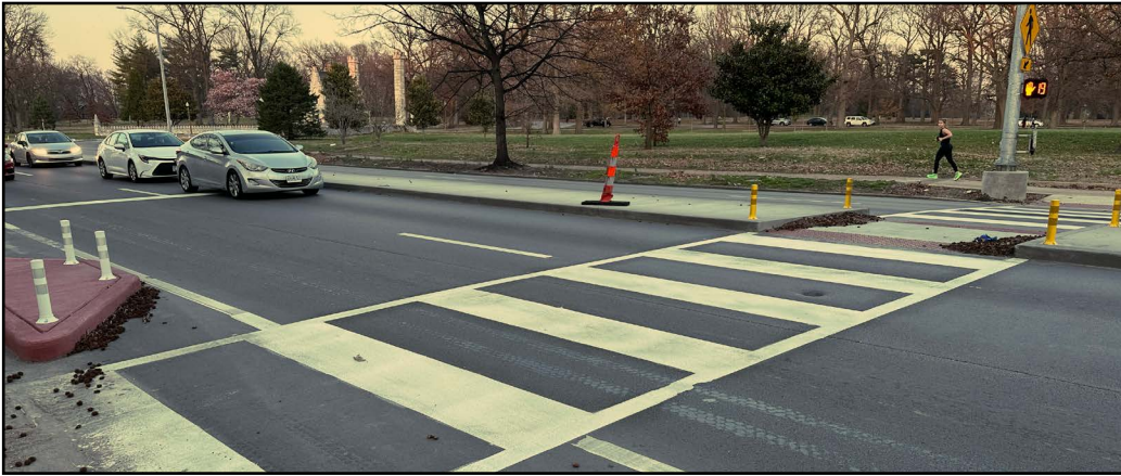
Left: Mid-block crossing and concrete median near Tower Grove Park Below: Intersection improvements that will link to future Christy Greenway extension
